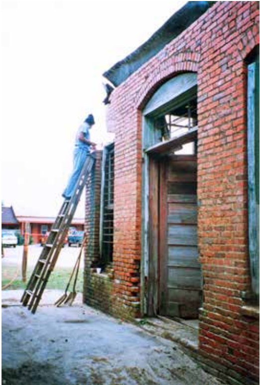
(top) Sections of the brick are removed and reset by inmate help from the Century Correctional Institute in Century, Florida.
