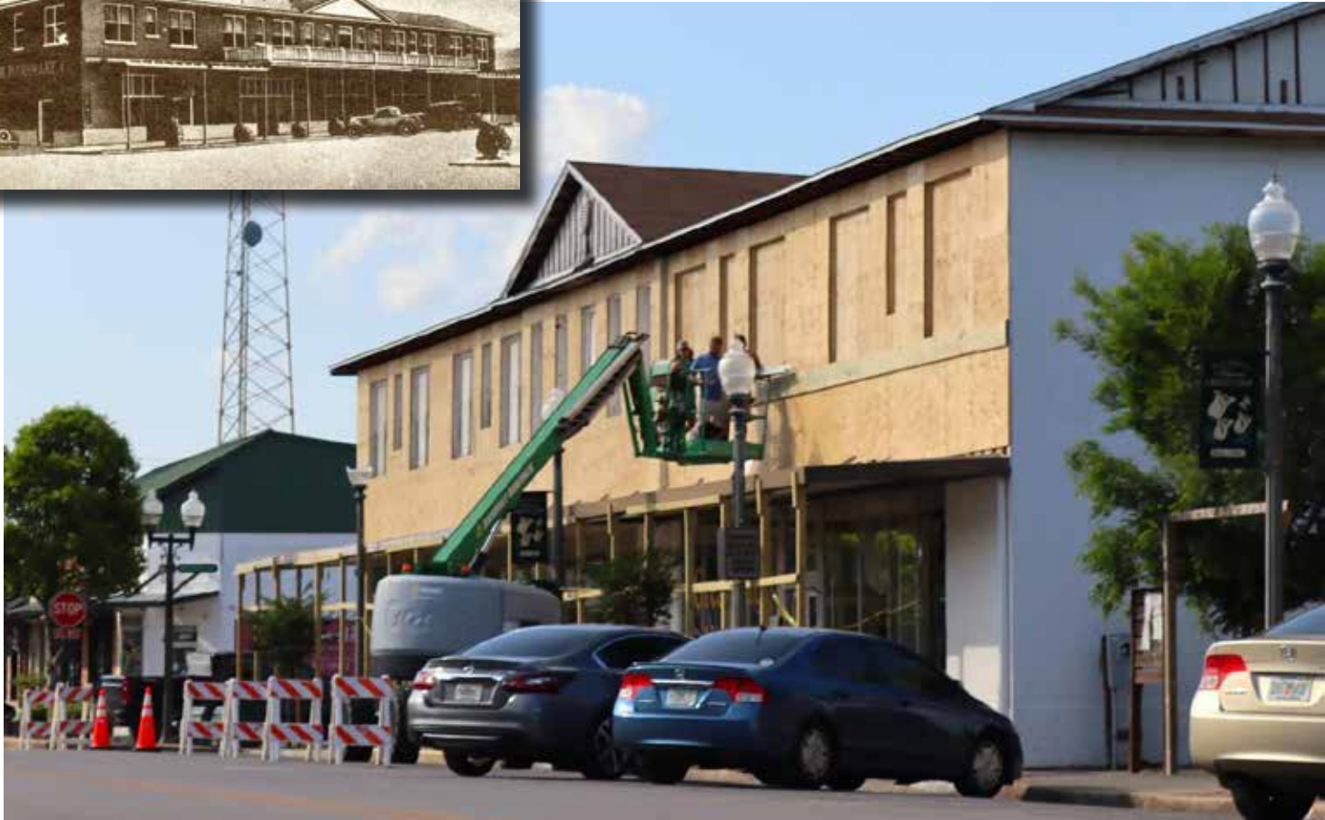
The removal of vinyl siding from the former Lamar and Hilton Hotel reveals the 1926 hotel's original upstairs front windows. The second floor will remain closed following the exterior renovation. (Photo by Brian Hughes) (inset) Crestview's Lamar Hotel was opened in 1926 on the site of the city's first business, the 1880s Powell Hotel. (Baker Block Museum photo)
