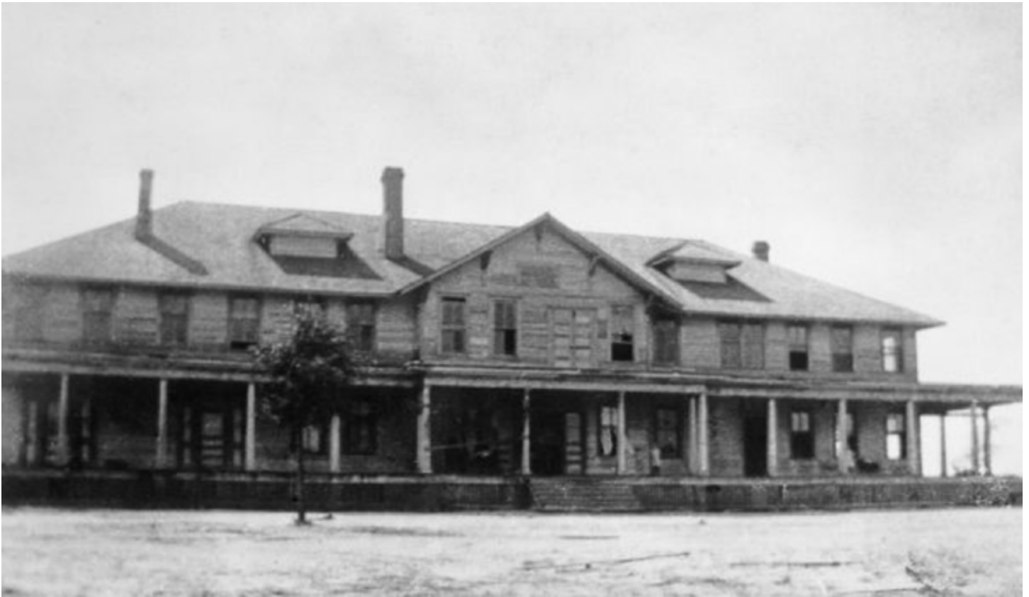
The Falco Hotel in an undated photo. The hotel was sold, dismantled, and the material was used to build the Covington Hotel in Opp, Alabama, around 1925.
